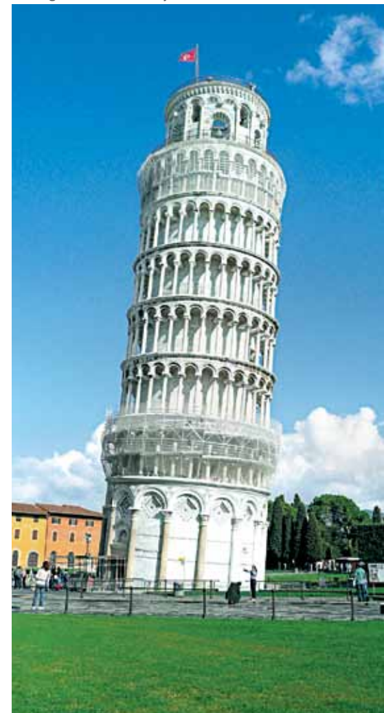
Leaning Tower of Pisa - Italy
