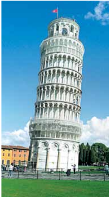
Leaning Tower of Pisa
